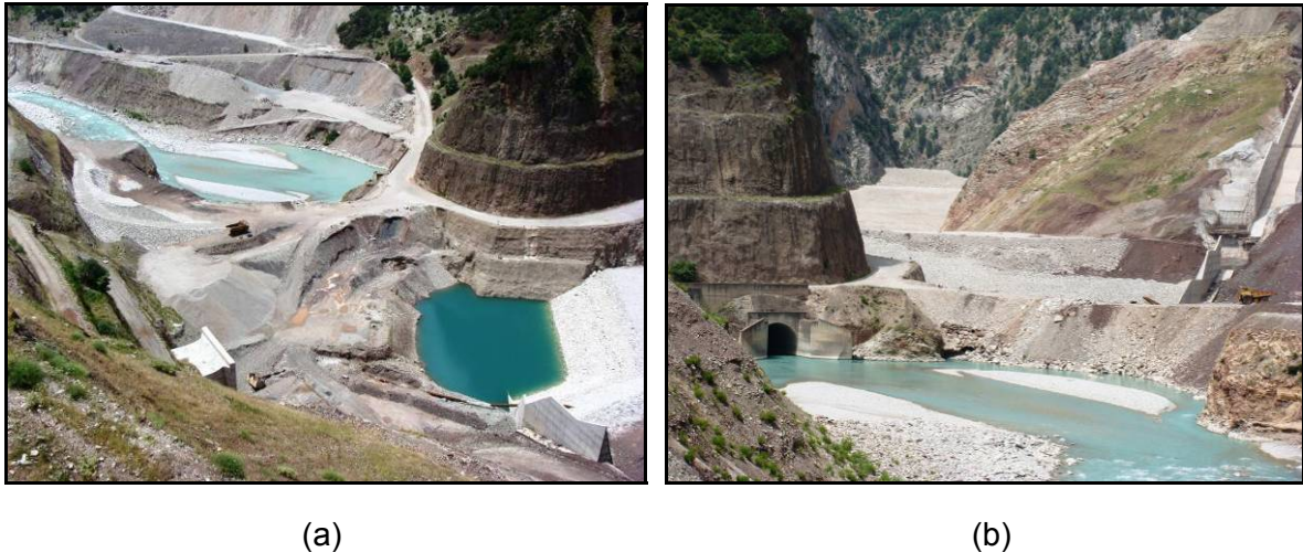
Photo. 4-6 – Downstream Cofferdam – (a) U/S view – (b) D/S view
