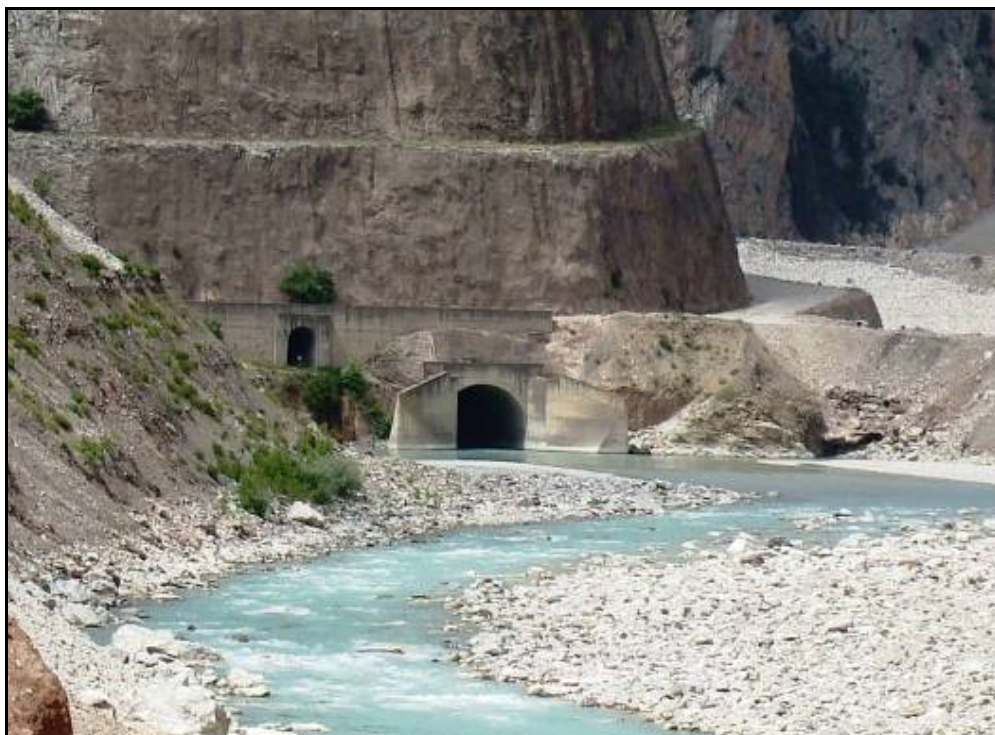
Photo. 4-2 - Acheloos Diversion Tunnel – Outlet Portal
