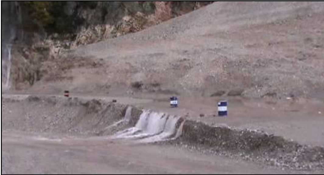
Photo. 6-6 - 2009 Flood - Water flow over the crest of the diaphragm wall.
