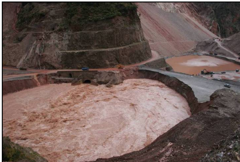
Photo. 6-2 – 2009 Flood: Outlet of Acheloos Diversion Tunnel – Erosion of cofferdam
