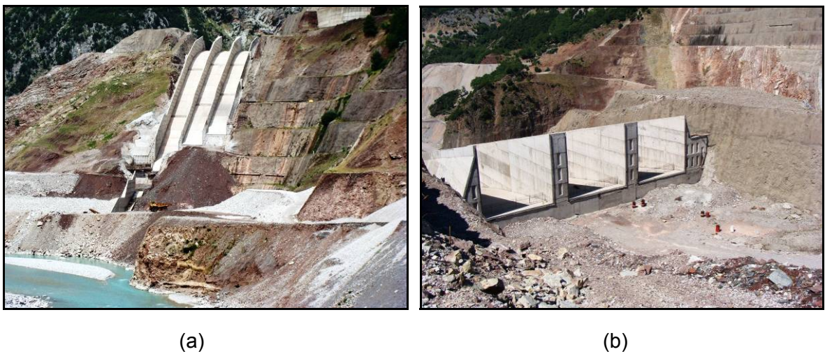
Photo. 4-10 – Spillway – (a): Three Channel Chute, (b): Upstream View of Channels
