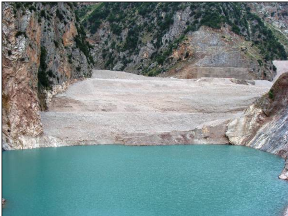
Photo. 4-7 - Upstream Dam Shell – View from D/S
