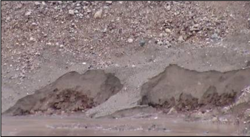
Photo. 6-4 - Piping and water flow above the crest of the diaphragm wall
