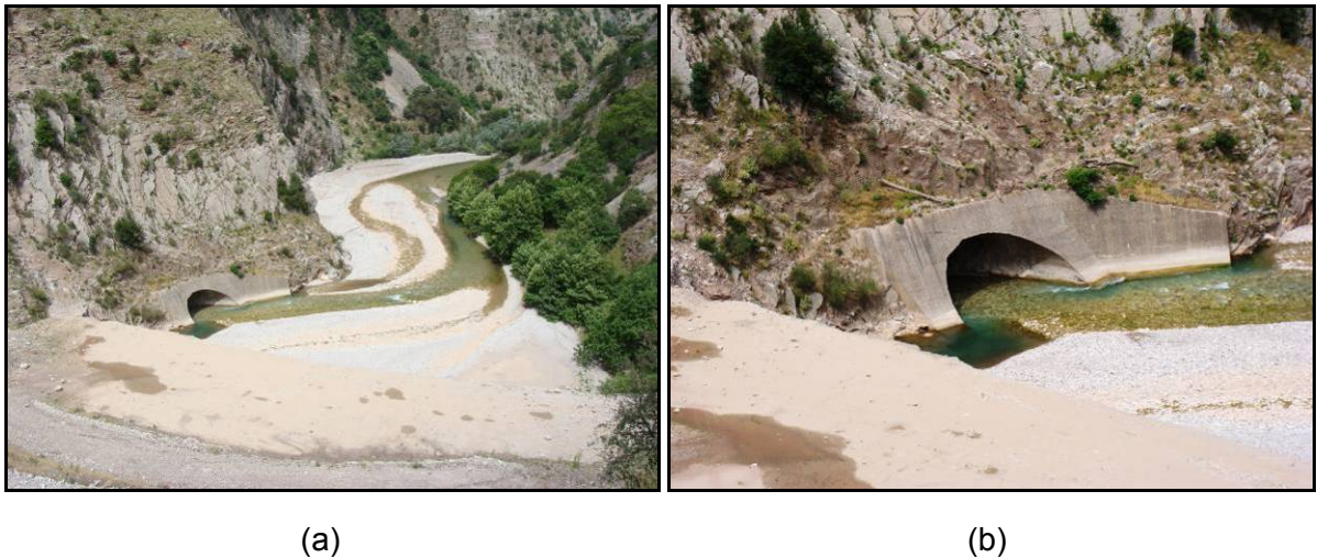
Photo. 4-3 – Koubourjiannitikos Diversion Tunnel – Inlet portal half filled with river sediments
