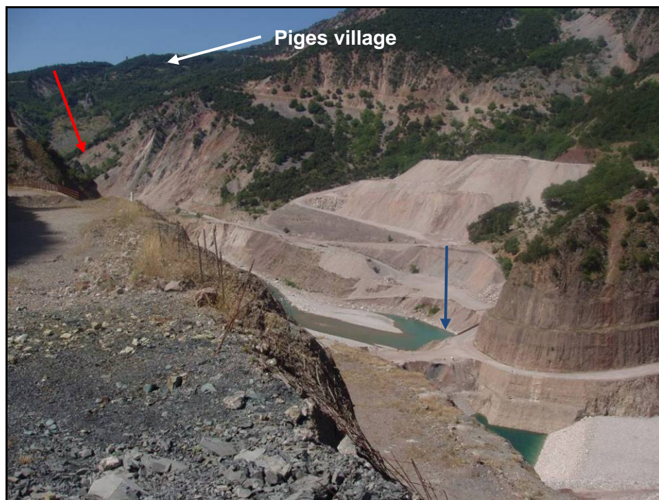
Photo. 5-6 - View of the downstream area. The exit of Acheloos diversion tunnel is shown (blue arrow), as well as Piges village and the 2003 landslide at the background (red arrow).
