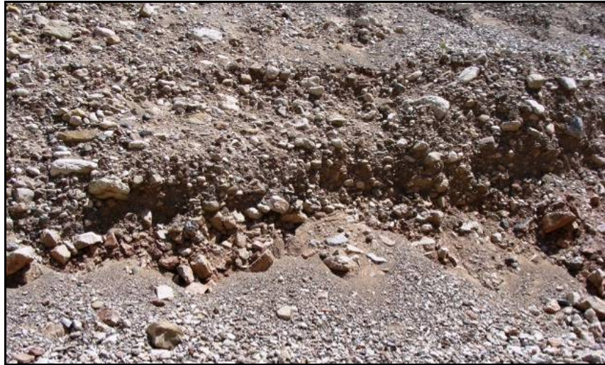
Photo. 6-7 – Formation of open gravels after washing of fines from dam shell
