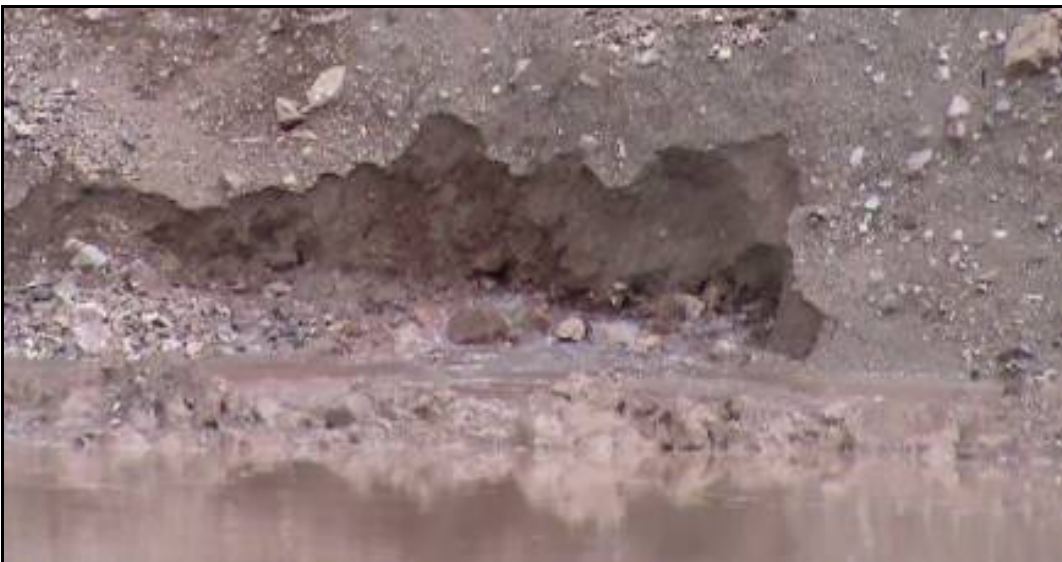
Photo. 6-5 - Piping and water flow above the crest of the diaphragm wall
