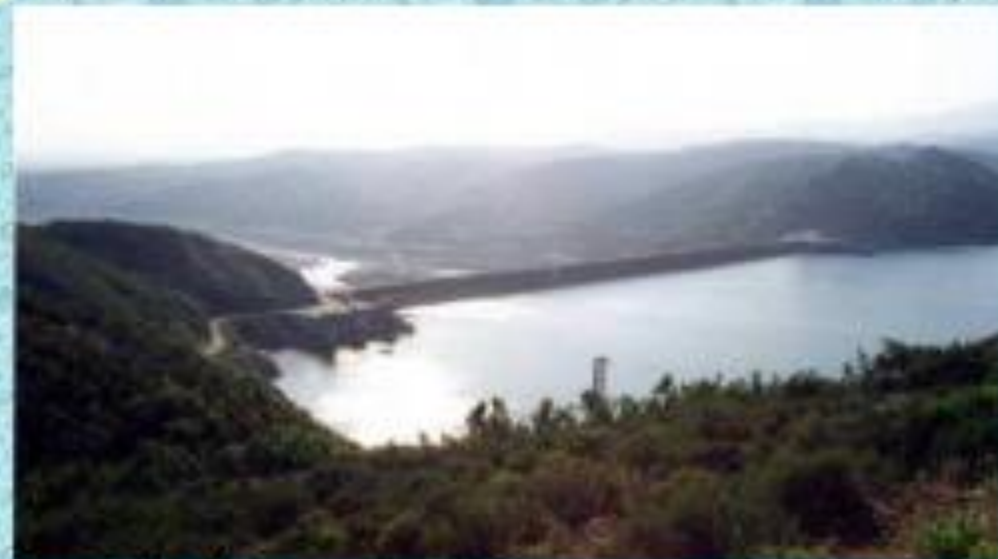
Dam construction in Greece
